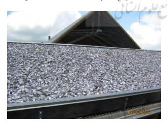
Fig.13: Use of mussel-shells in roofs of Munksogaard (Source: Loux,2011)
